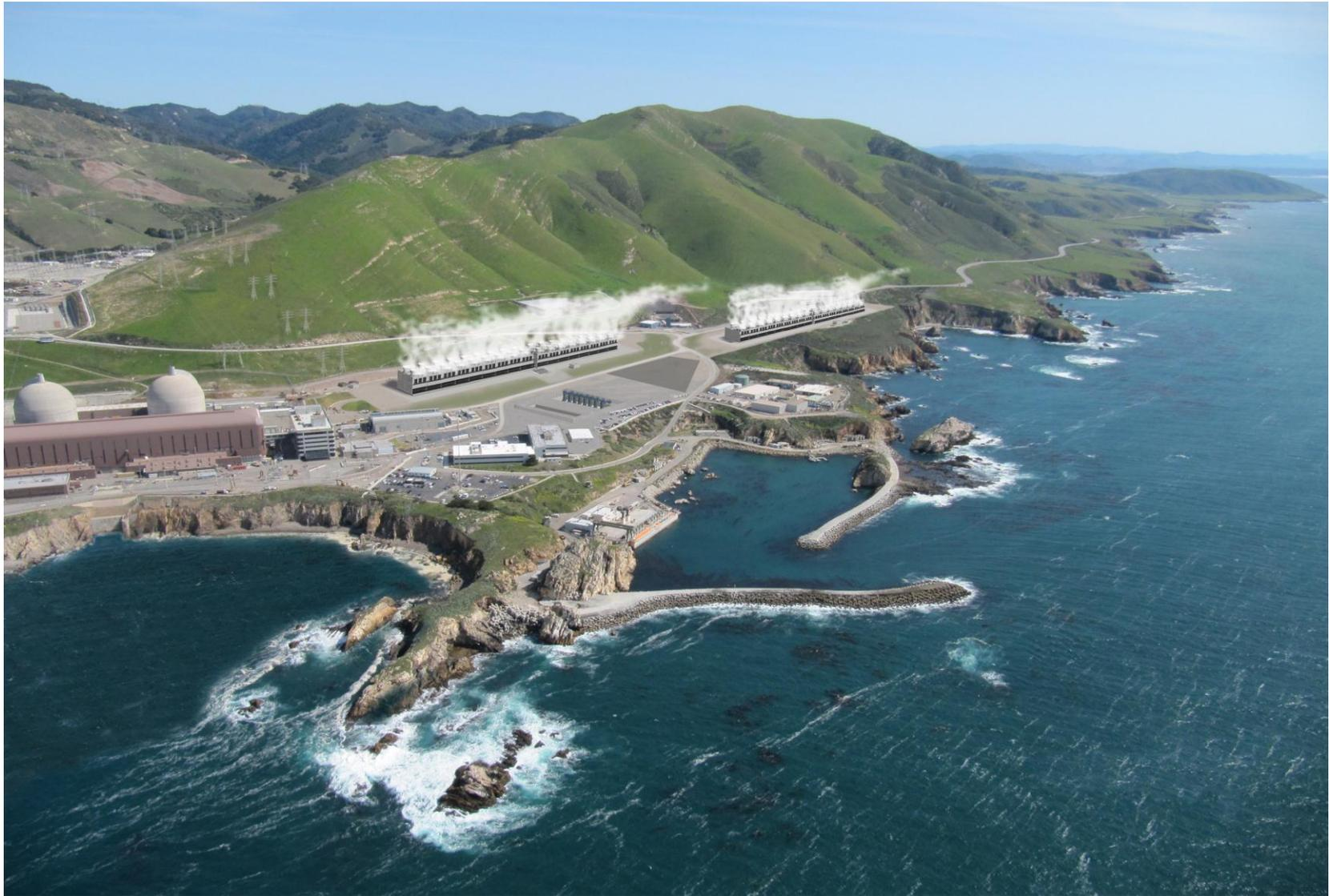
Figure 1.1-2. 34-Cell ClearSky Wet Mechanical Cooling Tower
