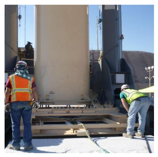
This picture shows the spotters, those are the people in the lift baskets, pulling the slings through the sheaths on the vertical cask transporter crossbeam. The important-to-safety yellow slings are connected to the canister through lift cleats in the shield cone and anchored to the vertical cask transporter. (Ex. 4, p. 7)
