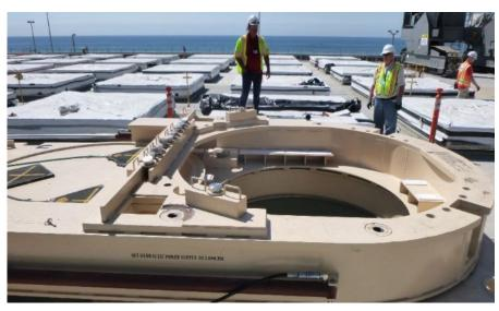
This photo shows the vertical cask transporter being aligned to the mating device, the vertical cask transporter is positioned over the mating device, properly aligned, and then they're bolted together. The mating device door is closed during this process. (Ex. 4, p. 7)
