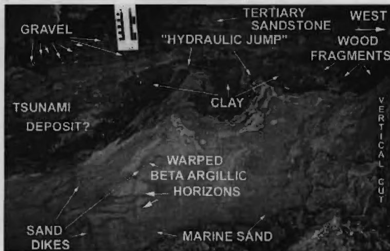
Fig. 30. View looking south of a storm drain trench wall cut into a coastal terrace exposing possible tsunami deposits at Carlsbad, California (15.54 m el. MSL). Note: Exposed are highly disturbed, contorted, chaotic, turbid sediments and debris overlying liquefied and dragged Bt horizons resting on a Tertiary sandstone abrasion platform. The upper half of this exposure interpreted as tsunamigenic in origin, for it also displays a distinct “hydraulic jump”, markedly different from documented paleoliquefaction features documented elsewhere.
