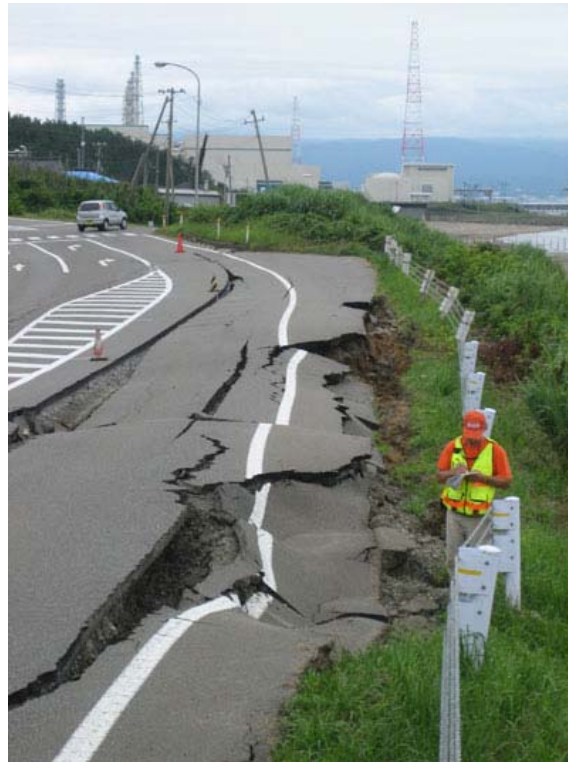
Figure 23: Coastal damage adjacent to the Kashiwazaki-Kariwa Nuclear Power Station 309
