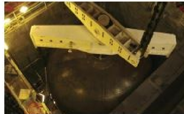
The RSG is lifted onto a purpose-built platform, slid into the building, and then set into its final position by the containment vessel's internal crane.
