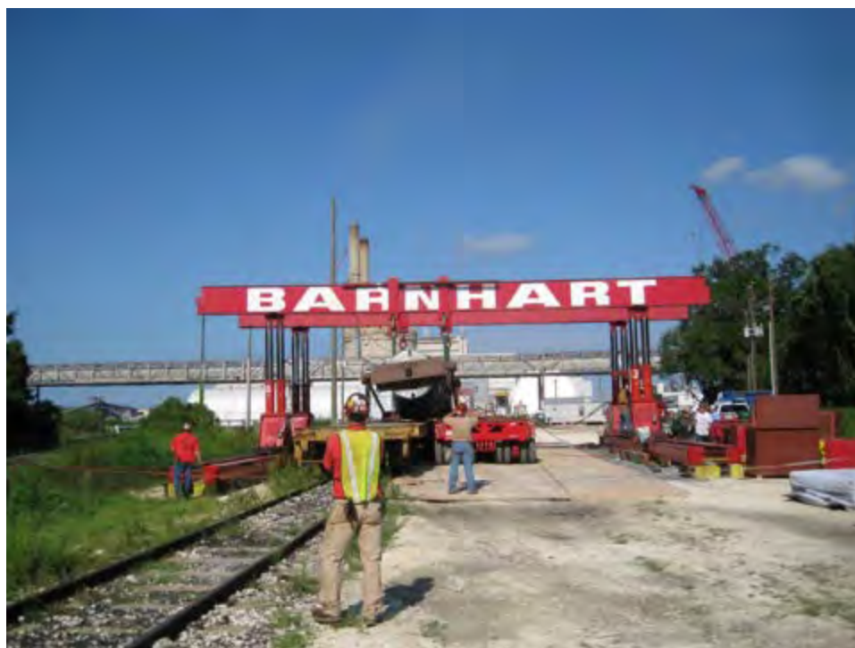
Figure 2-183. Generator Rotor Being Unloaded at the Crystal River Site (2009)
