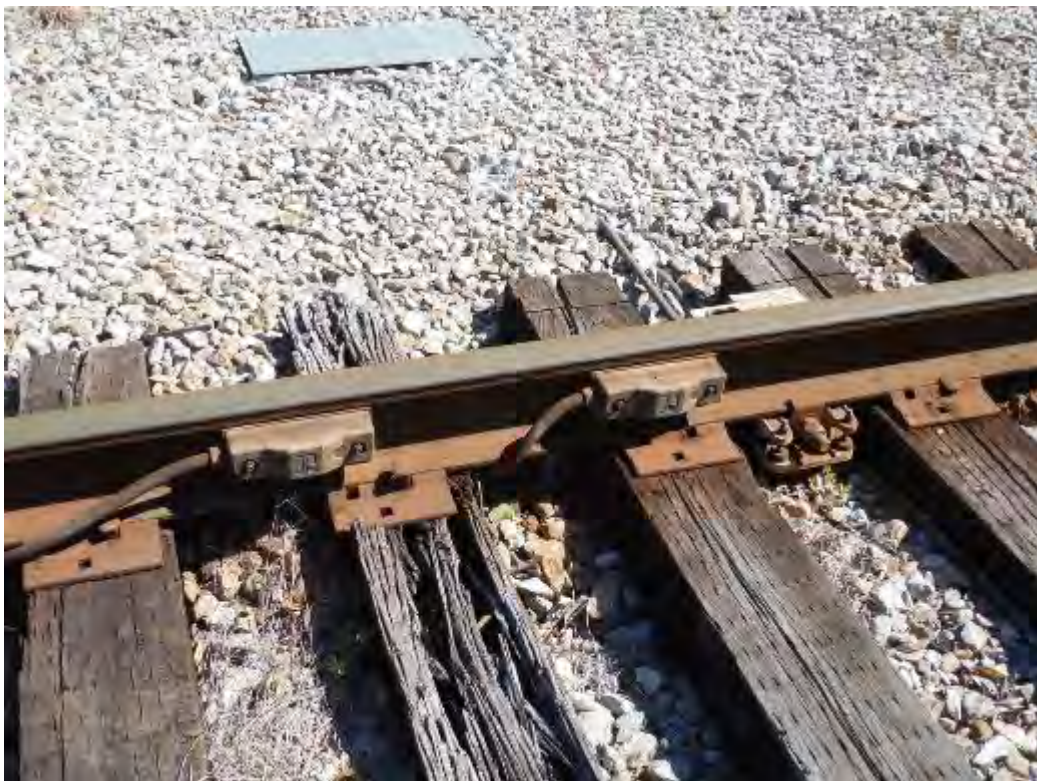
Figure 2-175. Wheel Detectors on Florida Northern Railroad (2015)
