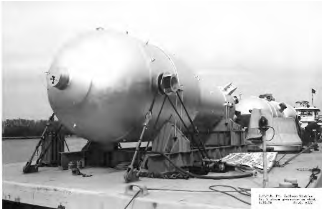
Figure 2-364. Steam Generators Being Shipped by Barge During Construction
