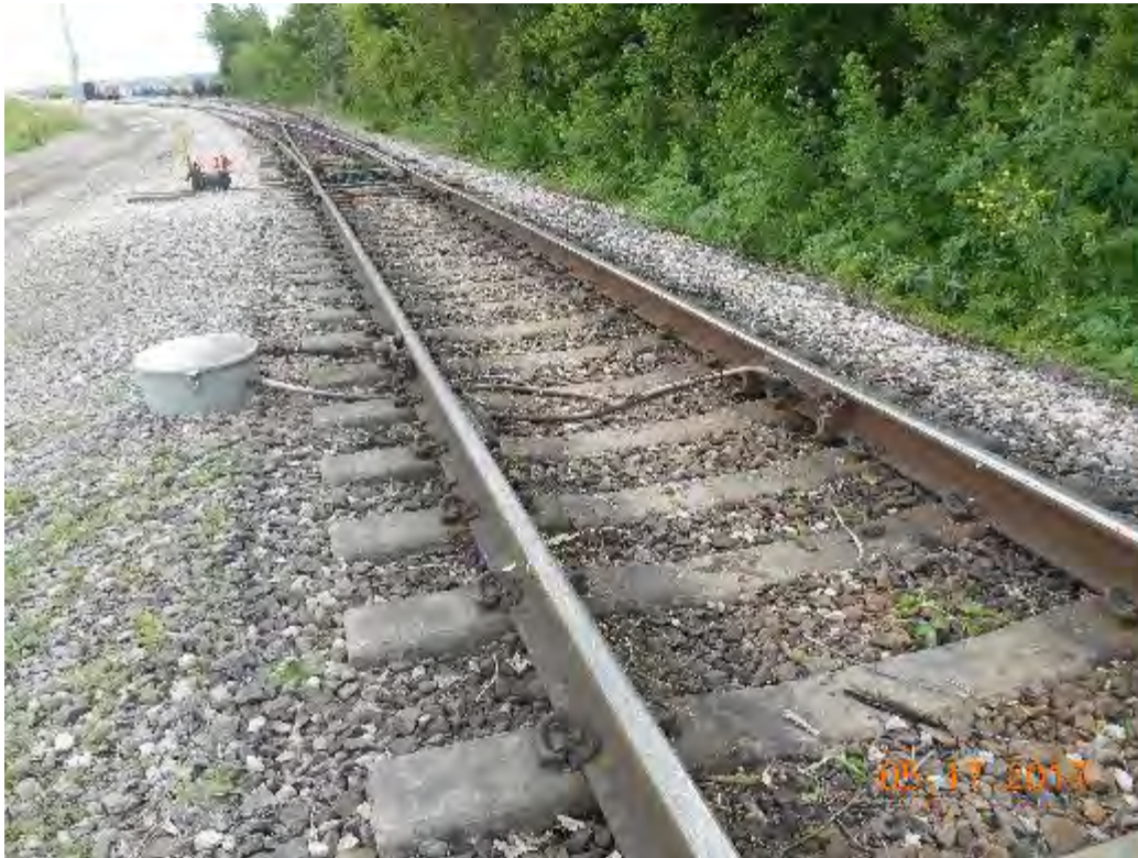
Figure 2-350. Derailer and Greaser on Cargill Industrial Spur (2017)
