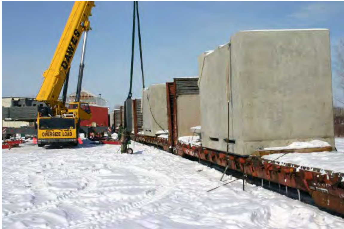
Figure 2-222. Horizontal Storage Module Transloading at Bellevue Location (2008)
