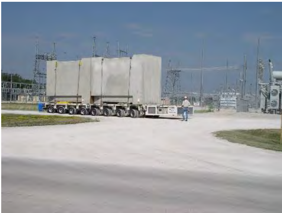
Figure 2-358. Horizontal Storage Modules Being Moved on Haul Road to Independent Spent Fuel Storage Installation
