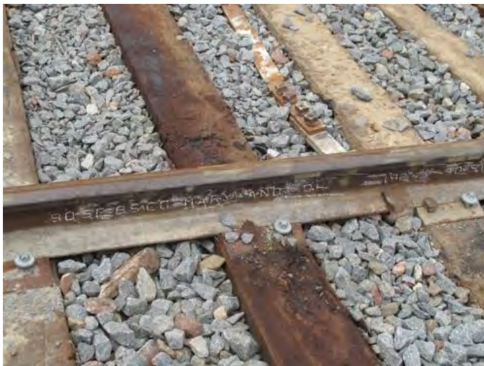
Figure B-60. Site Lead 90-lb. Rail (2015)
