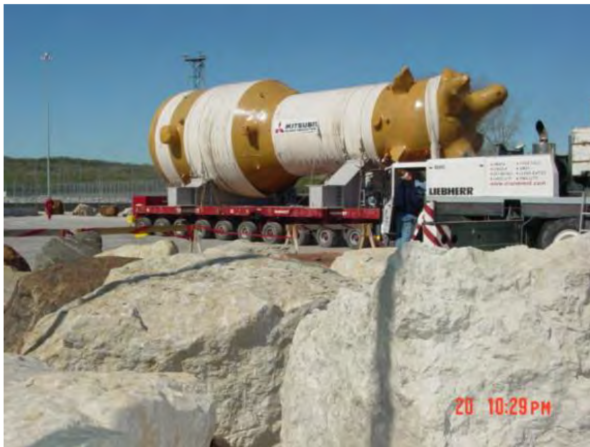
Figure 2-370. Steam Generator on Transporter After Unloading (2006)
