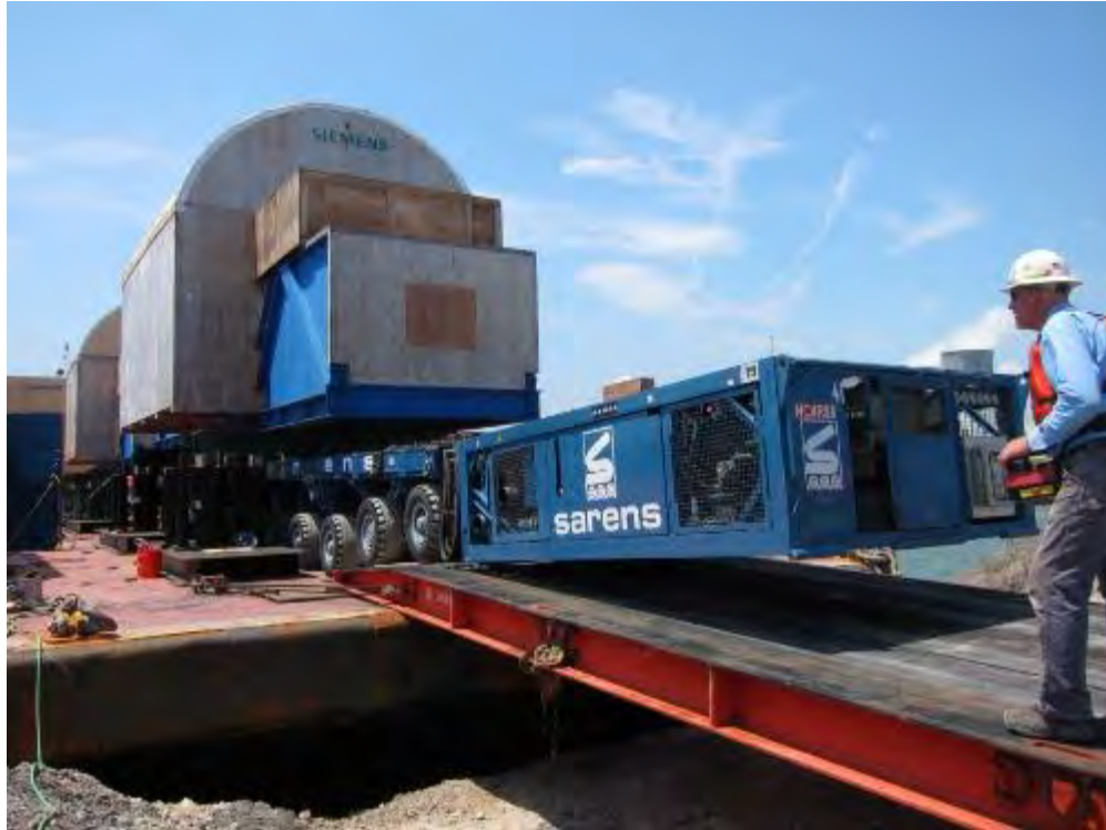
Figure 2-195. Turbine Components Being Unloaded Using Self-Propelled Modular Transporter (2012)
