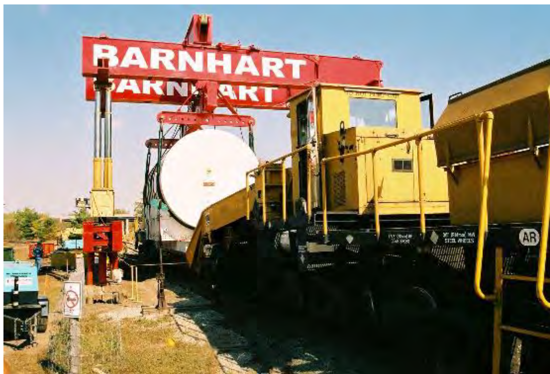
Figure 2-72. Transfer of Reactor Pressure Vessel onto ETMX1001 Railcar (2003)
