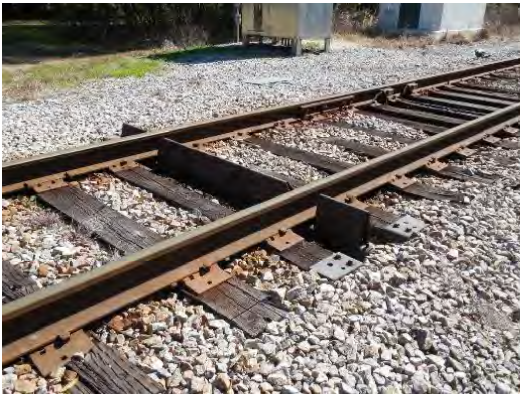
Figure 2-177. Dragging Equipment Detector on Florida Northern Railroad (2015)
