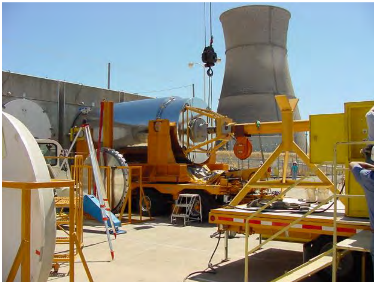
Figure 2-88. MP187 Transportation Cask and Hydraulic Ram Being Used to Load a Canister into a Horizontal Storage Module at Rancho Seco
