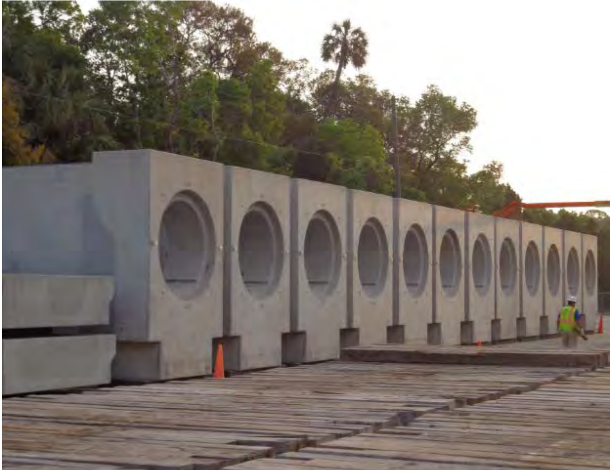
Figure 2-189. Horizontal Storage Modules at Nuclear Spur after Unloading (2015)
