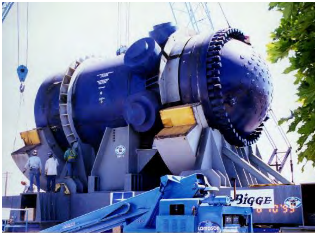
Figure 2-115. Trojan Reactor Pressure Vessel on Transport Cradle (1999)
