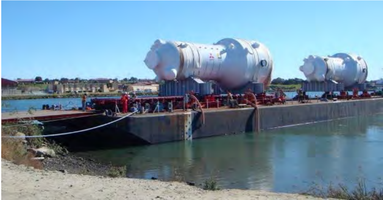
Figure 2-295. Offloading of Steam Generator on Goldhofer Trailer at Del Mar Boat Basin Bulkhead (2009)
