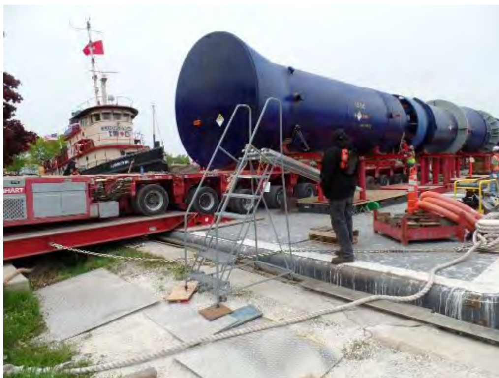
Figure 2-256. Fourth Steam Generator Moving onto Barge (2014)
