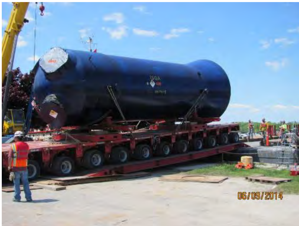
Figure 2-254. First Steam Generator on Goldhofer Trailer Moving onto Barge (2014)
