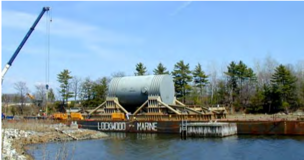
Figure 2-18. Maine Yankee Reactor Pressure Vessel Being Loaded onto Barge (2003)
