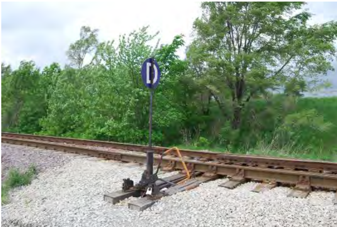
Figure 2-348. Derailer at Entrance to Cargill Industrial Spur (2017)
