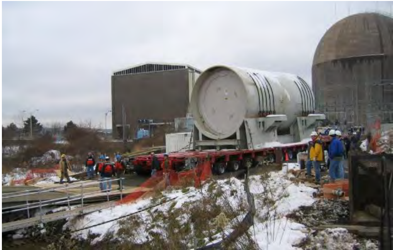
Figure 2-43. Connecticut Yankee Reactor Pressure Vessel Being Loaded onto Barge
