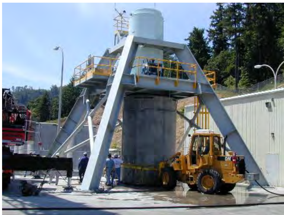
Figure 2-106. Trojan Transfer Station with Transfer Cask and TranStor Vertical Concrete Storage Overpack
