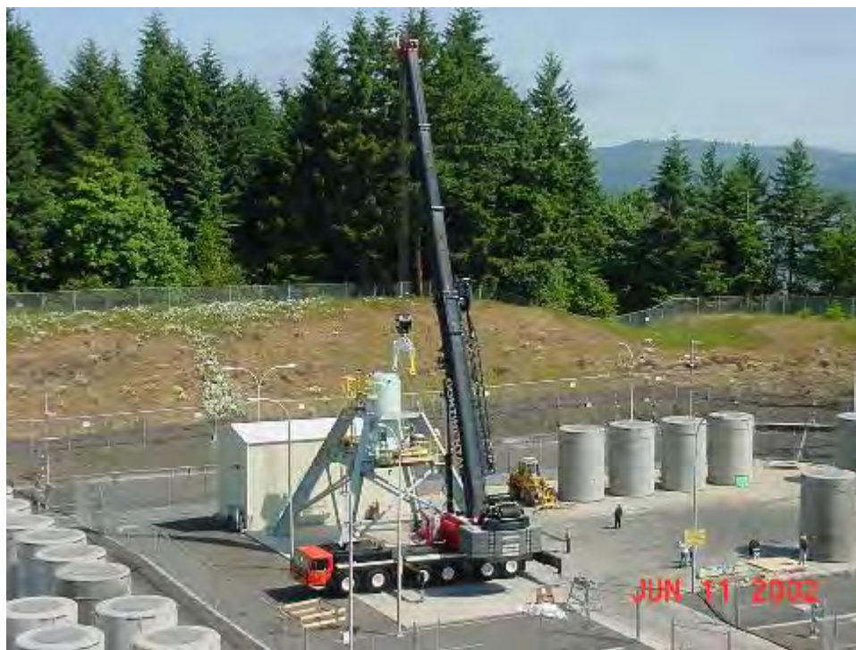
Figure 2-105. Trojan Transfer Station with Transfer Cask and Mobile Crane
