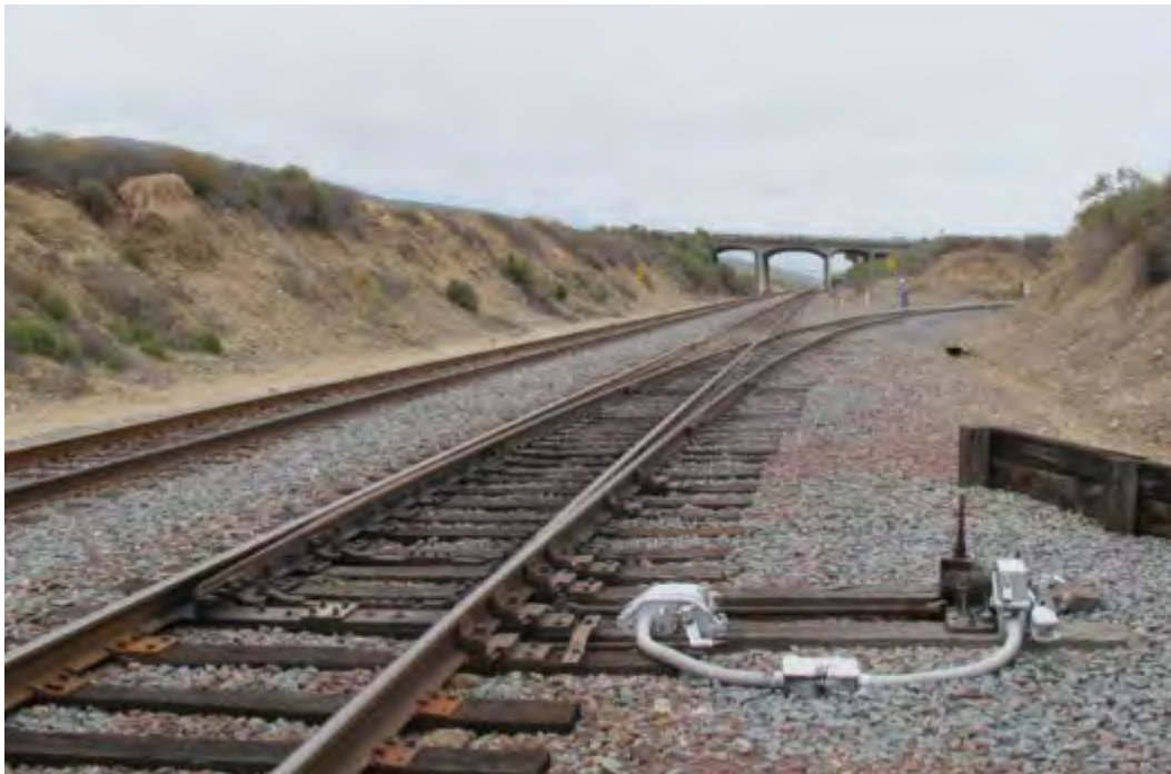
Figure B-56. Manually Operated, Timed Switch (2015)
