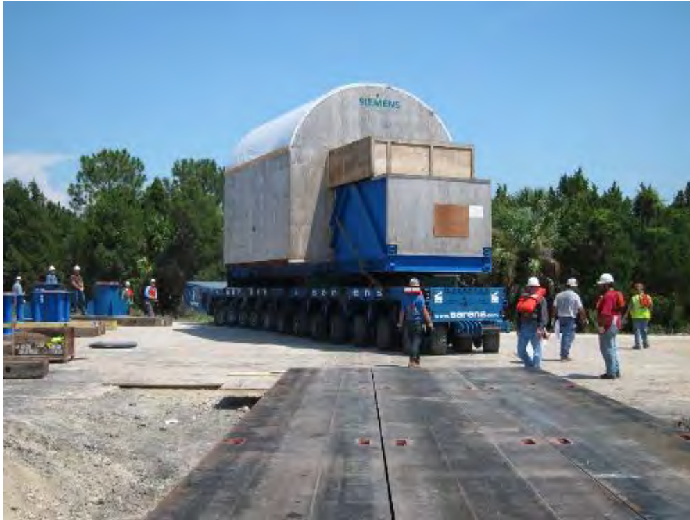
Figure 2-197. Turbine Components Fully Unloaded from Barge (2012)
