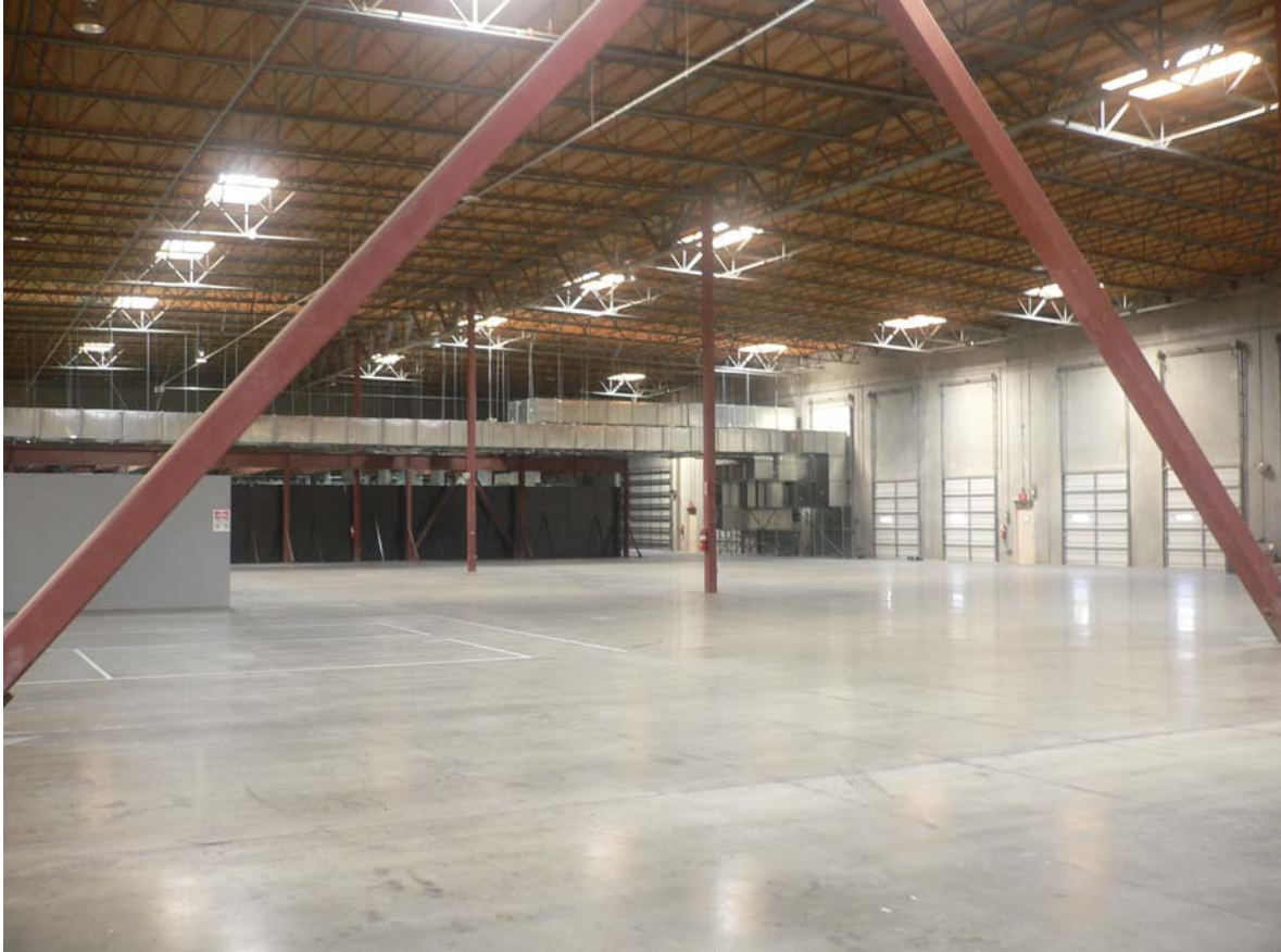
Photograph of Blackwater Facility
